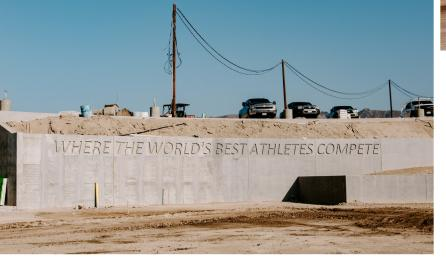
To prepare the site for the new Stadium, 680,000 cubic yards of soil were required to be relocated on campus or exported. After months of export operation with comprehensive dust management and SWPPP plans in place, while respecting truck trip limitations to minimize impact to local neighbors, the massive excavation was accomplished with zero campus and neighbor issues.
