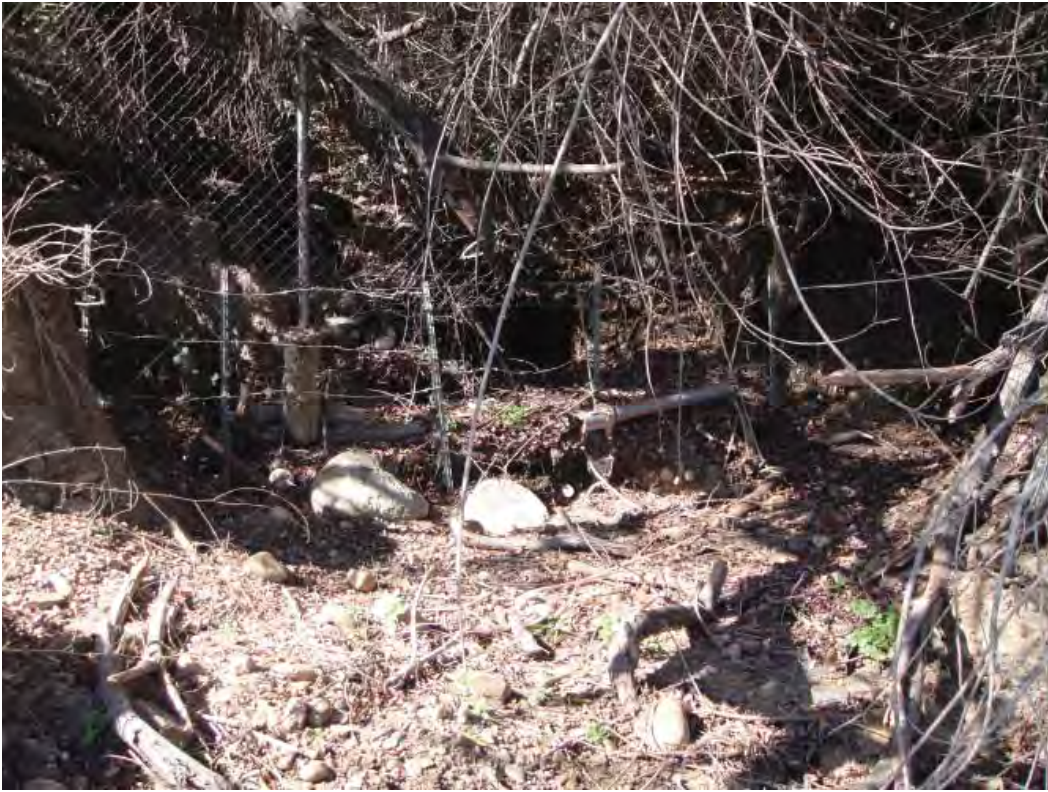
Northern drainage at western property boundary.
