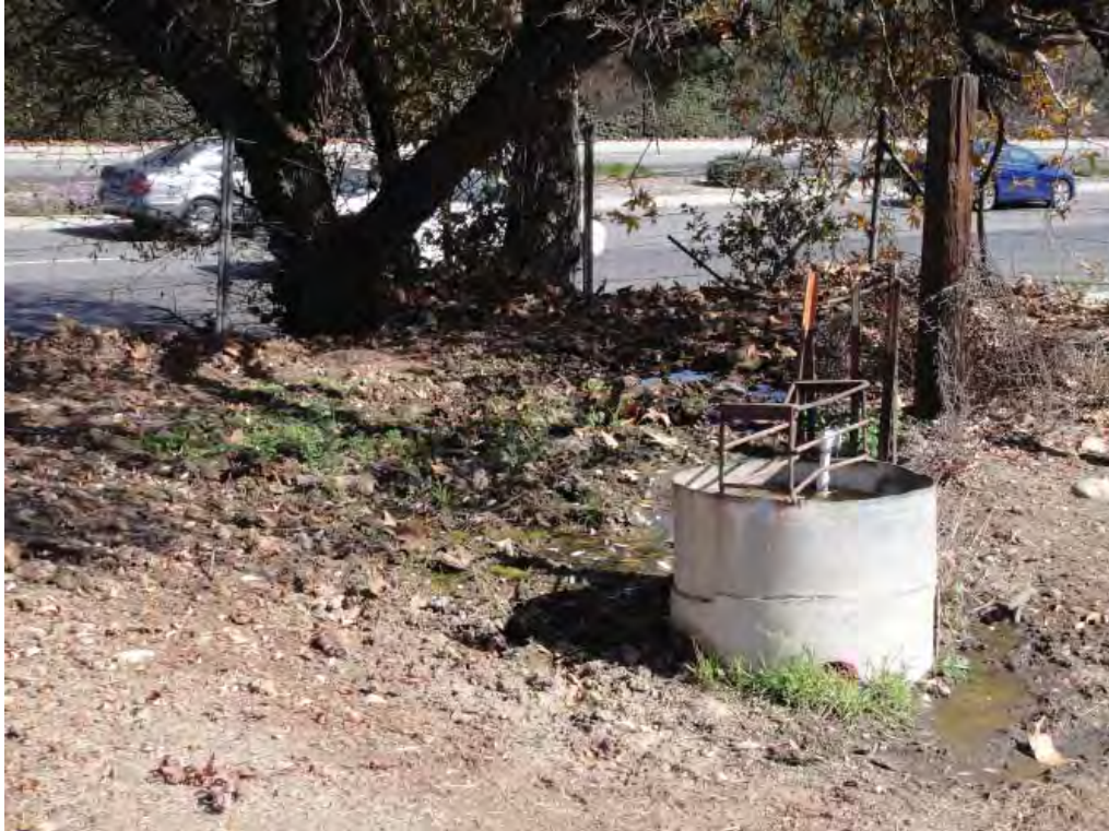
Leaky infrastructure near North Grand Avenue.
