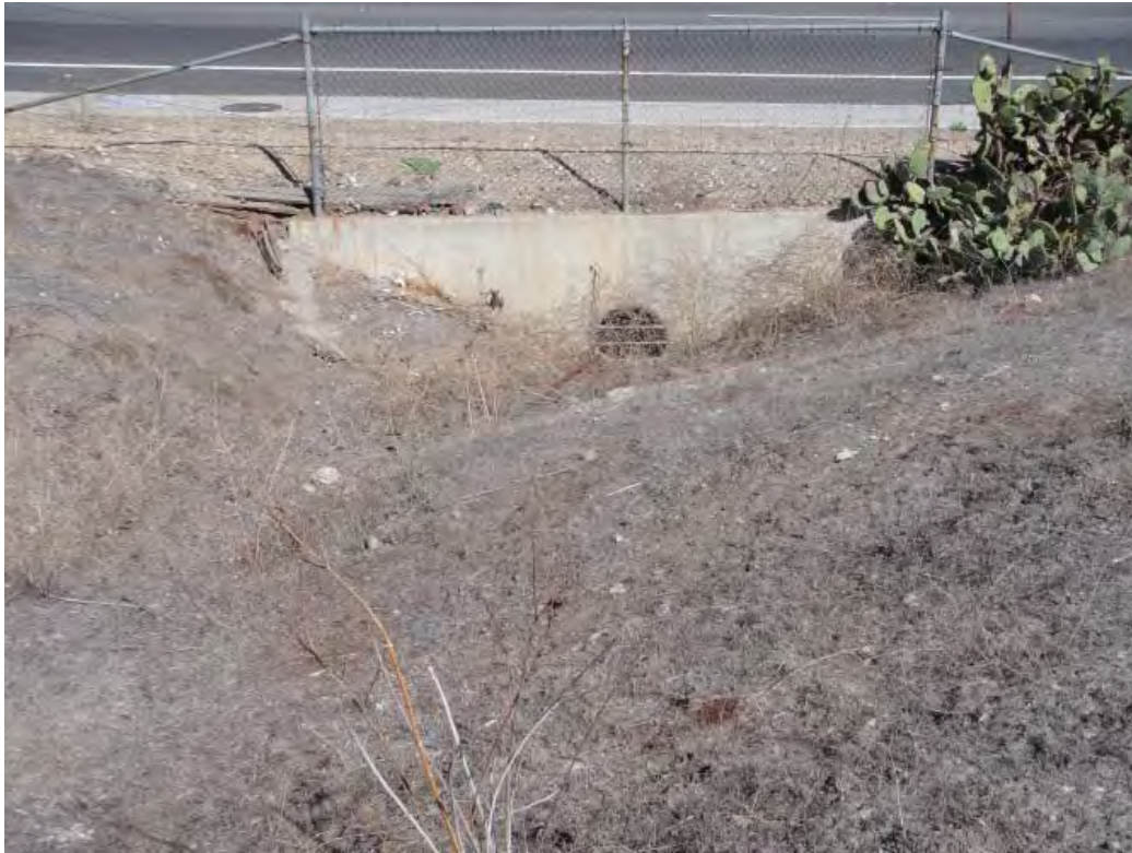
Southern drainage culvert inlet at North Grand Avenue.
