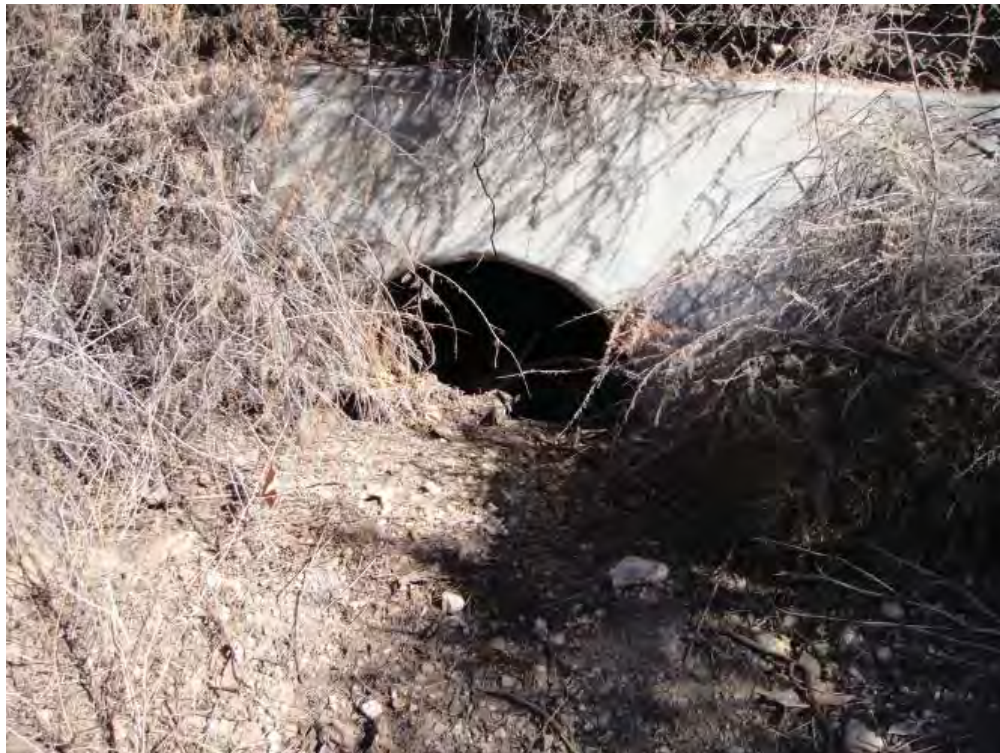
Northern drainage culvert inlet at North Grand Avenue.
