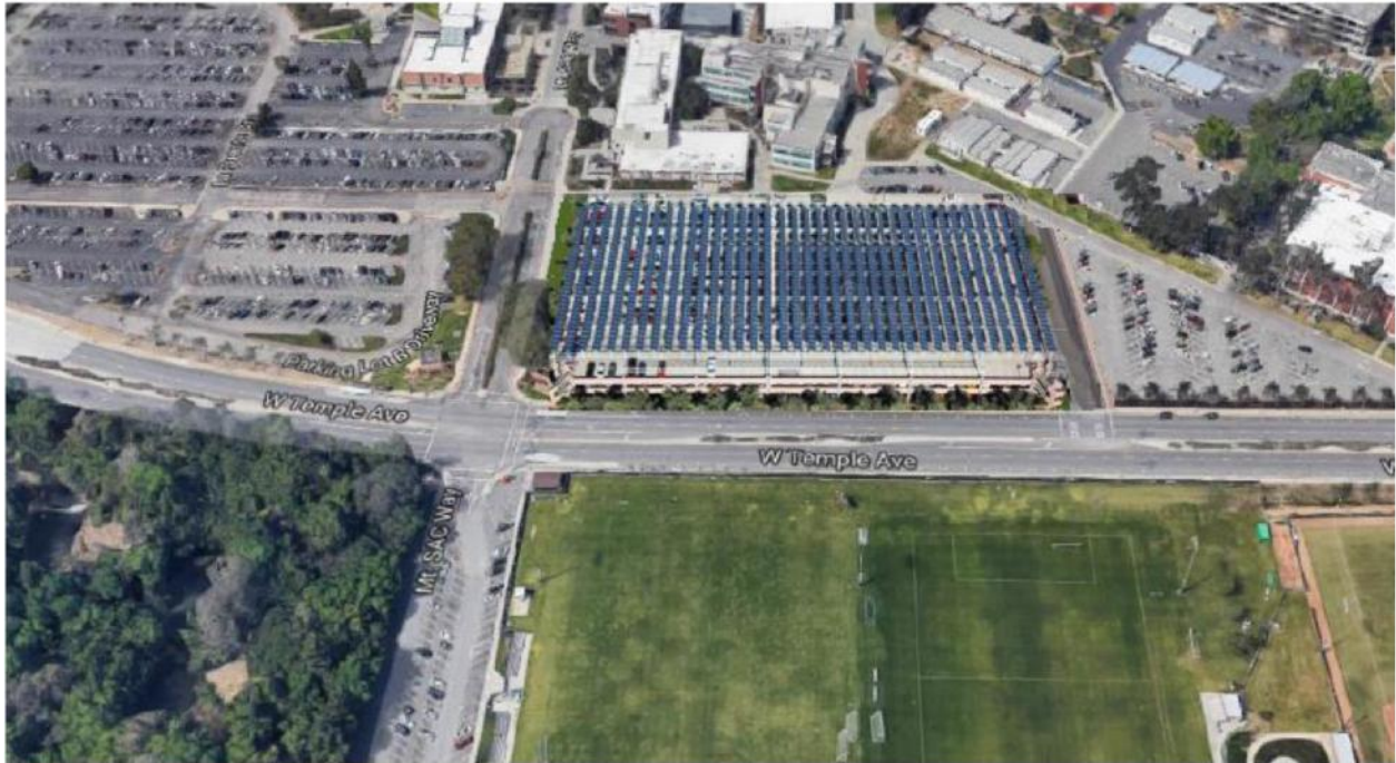
Depiction of Lot D Parking Structure with Solar Panel Canopies at Roof Level
