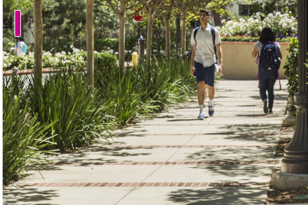
Concrete paving with brick accents.
