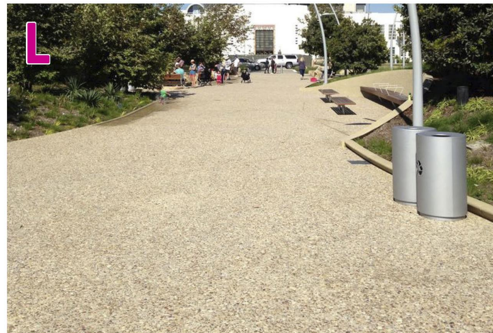
Lithocrete (exposed aggregate) concrete paving.
