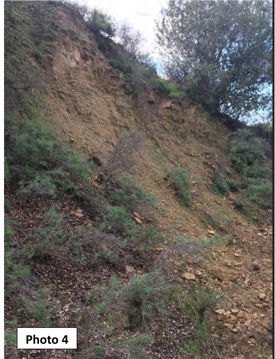
West Side of Landslide Escarpment (February 11, 2017)
