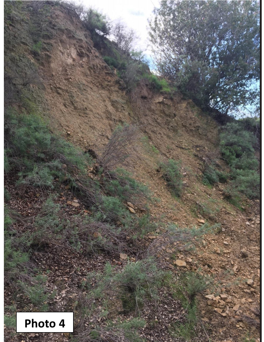
West Side of Landslide Escarpment (February 11, 2017)
