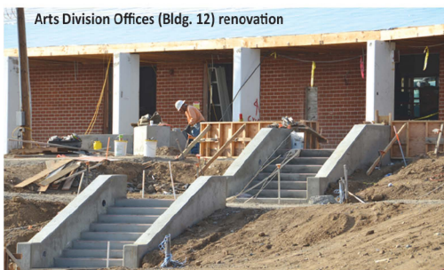
Arts Division Offices (Bldg. 12) renovation
