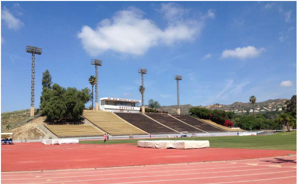
Hilmer Lodge Stadium (Condition as depicted in the May 2017 SEIR)
