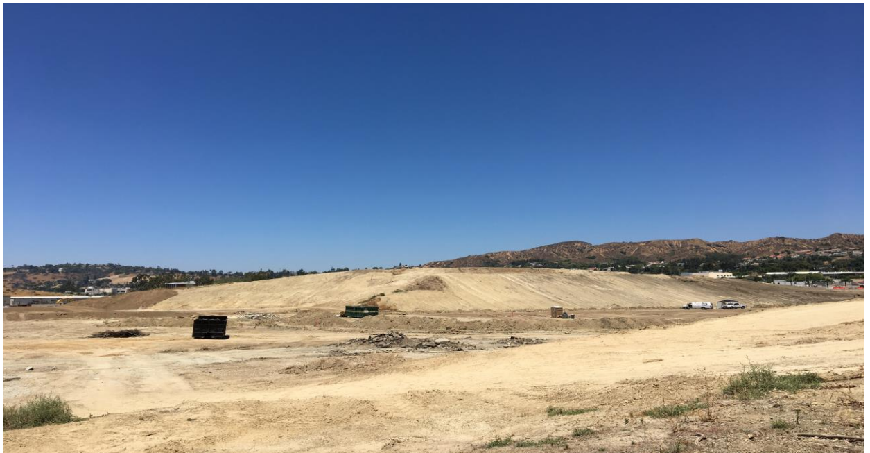
Hilmer Lodge Stadium (Existing Condition July 2017)
