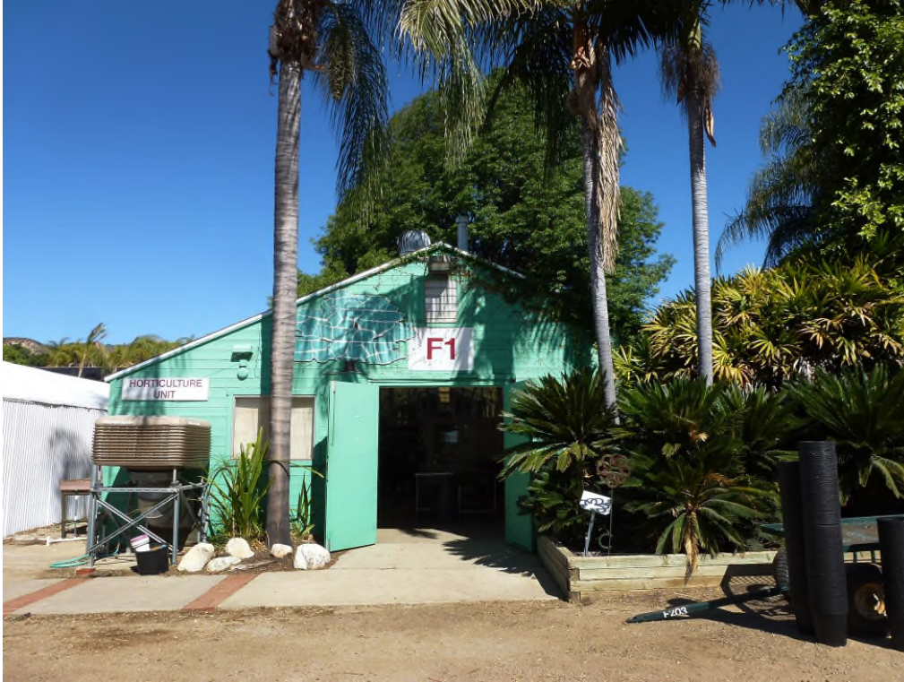
Figure 26. View of the south façade of Building F1.
