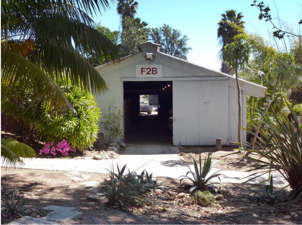
Figure 28. View of the west façade of Building F2B.
