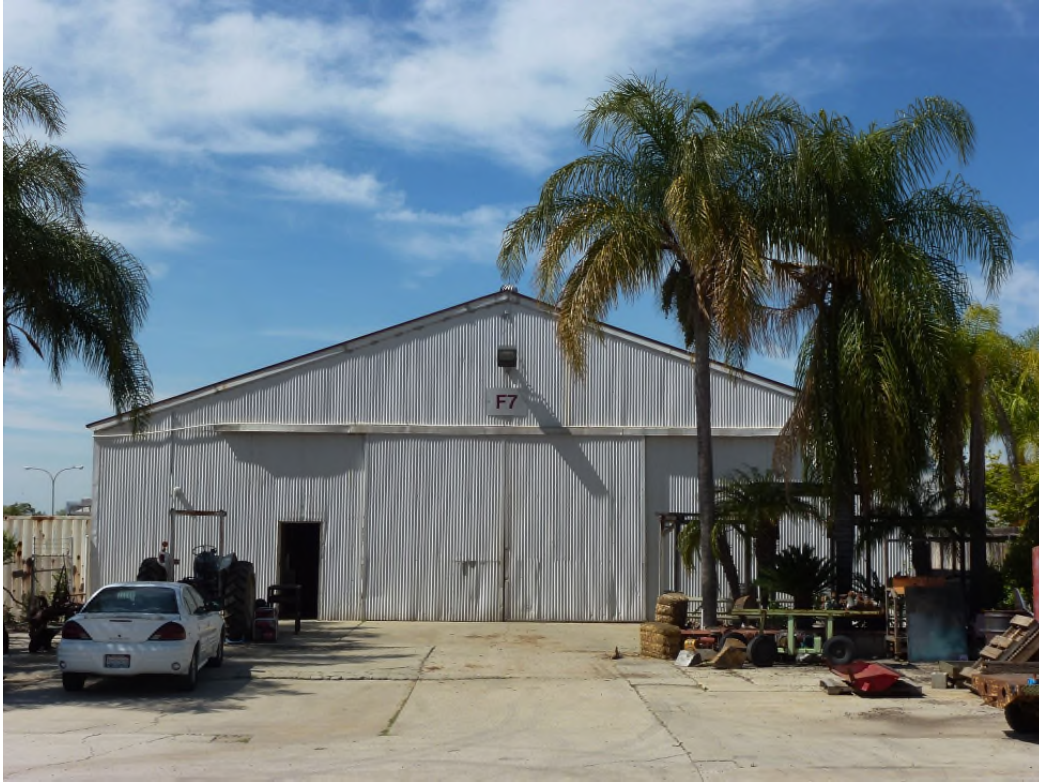
Figure 33. View of the east façade of Building F7.
