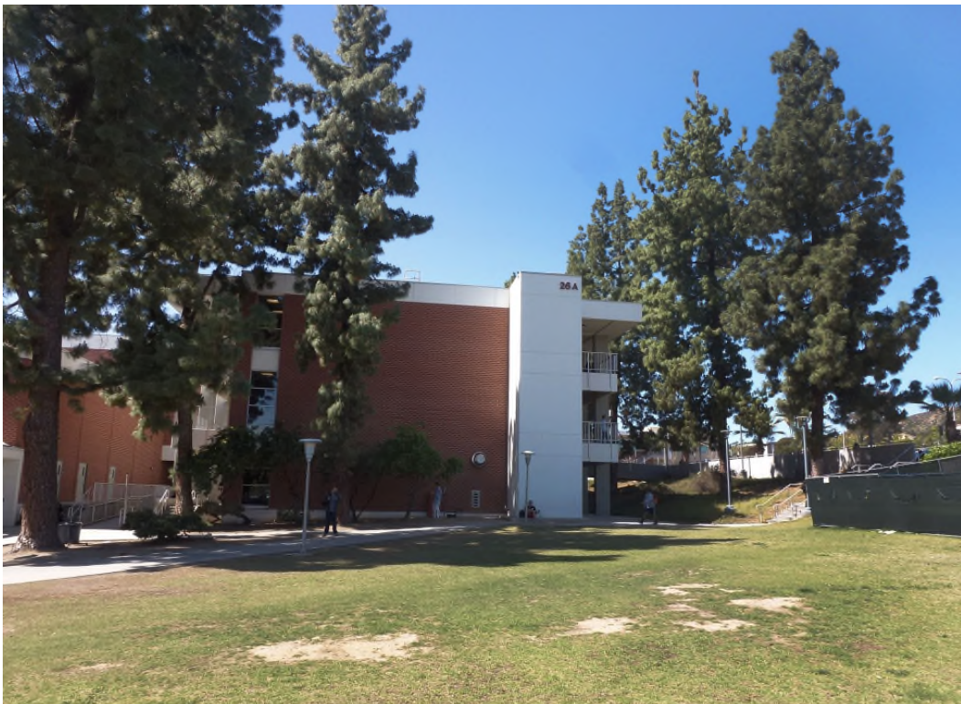
Figure 19. View of the east façade of Building 26A.
