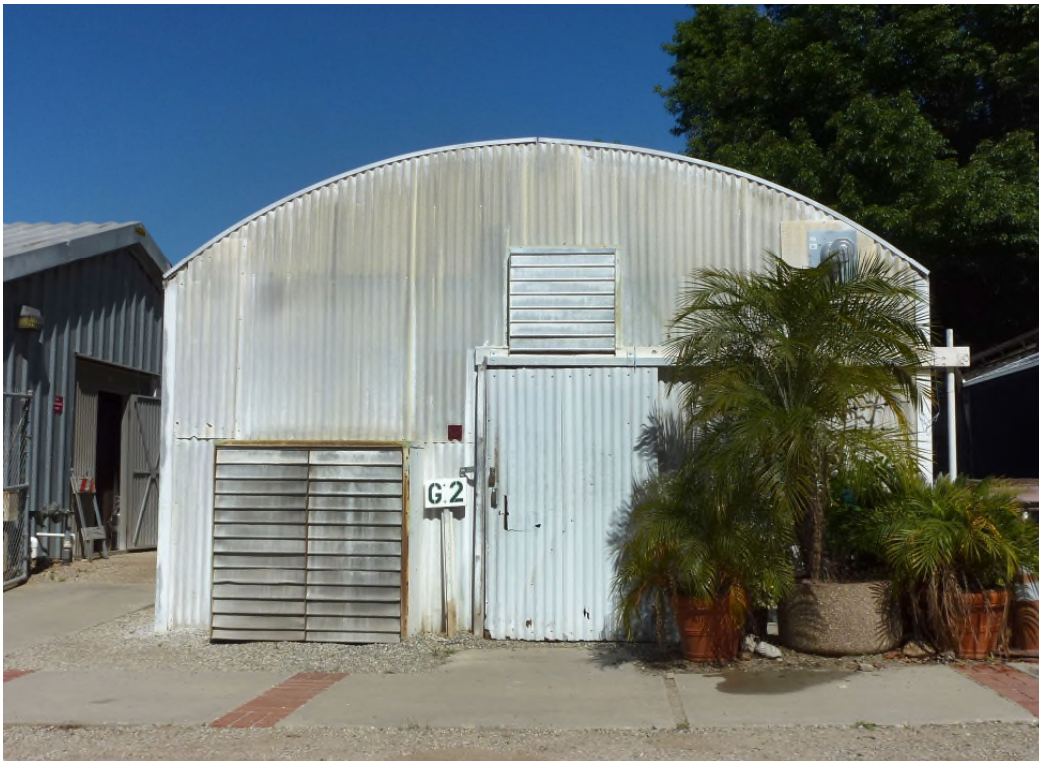
Figure 34. View of the south façade of Building G2.
