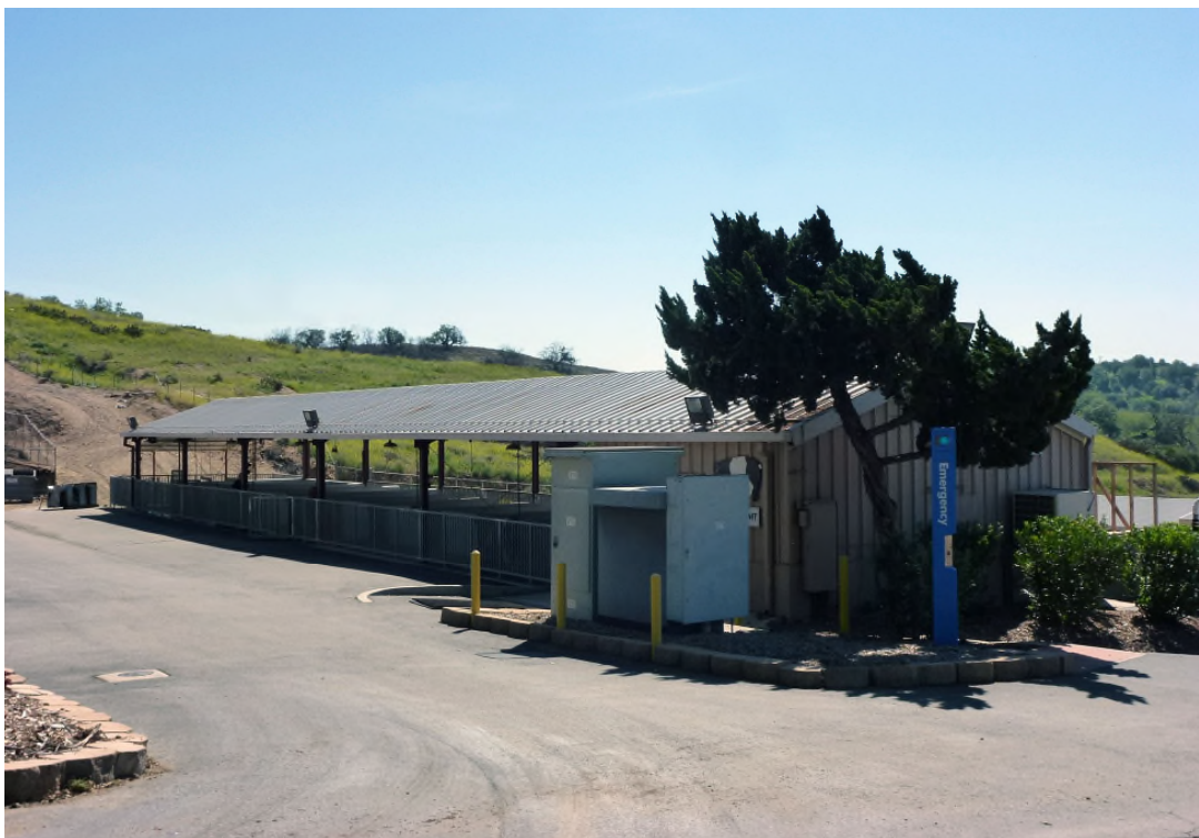
Figure 30. Oblique view of the north and west façades of Building F4A.
