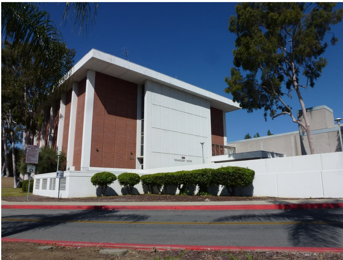
Figure 23. Oblique view of south and east facades of Building 28 A/B.
