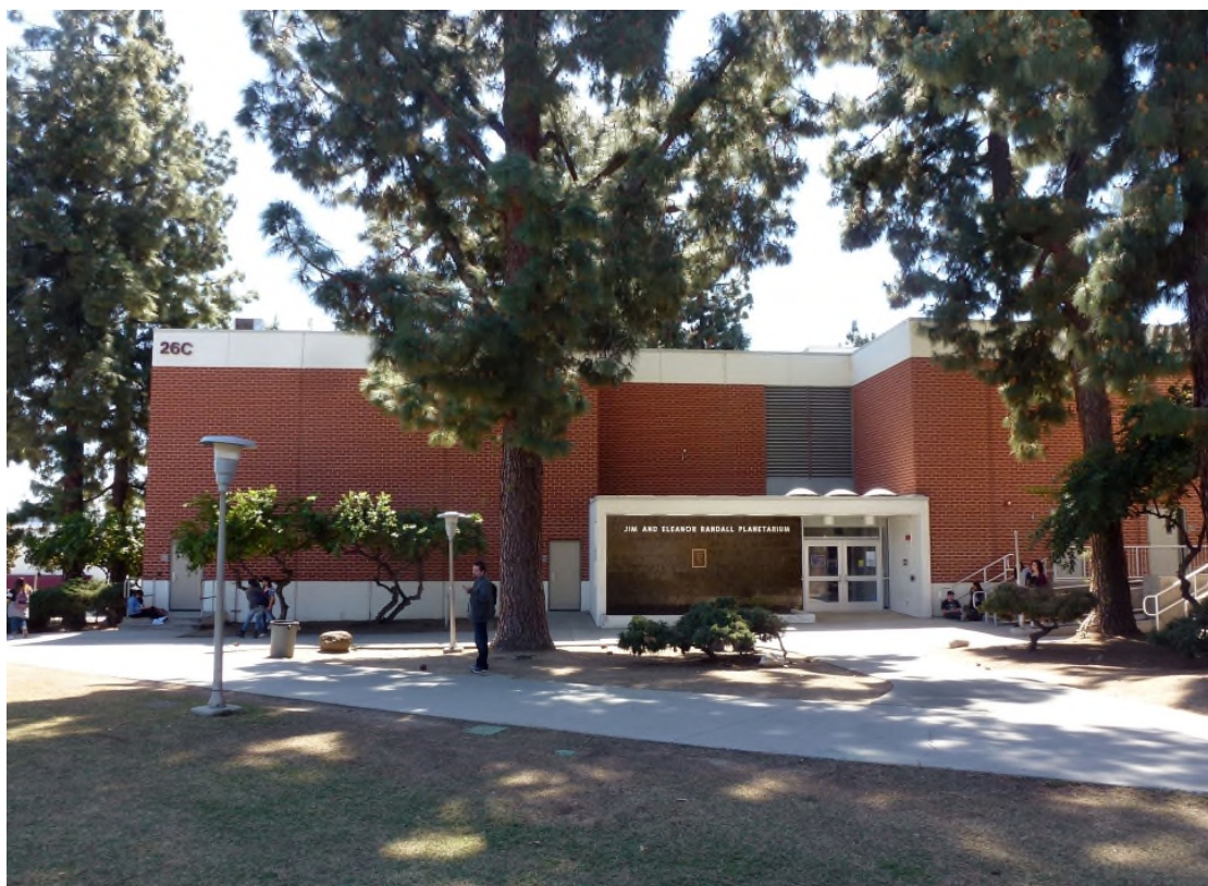
Figure 22. View of the south façade entrance of Building 26C.
