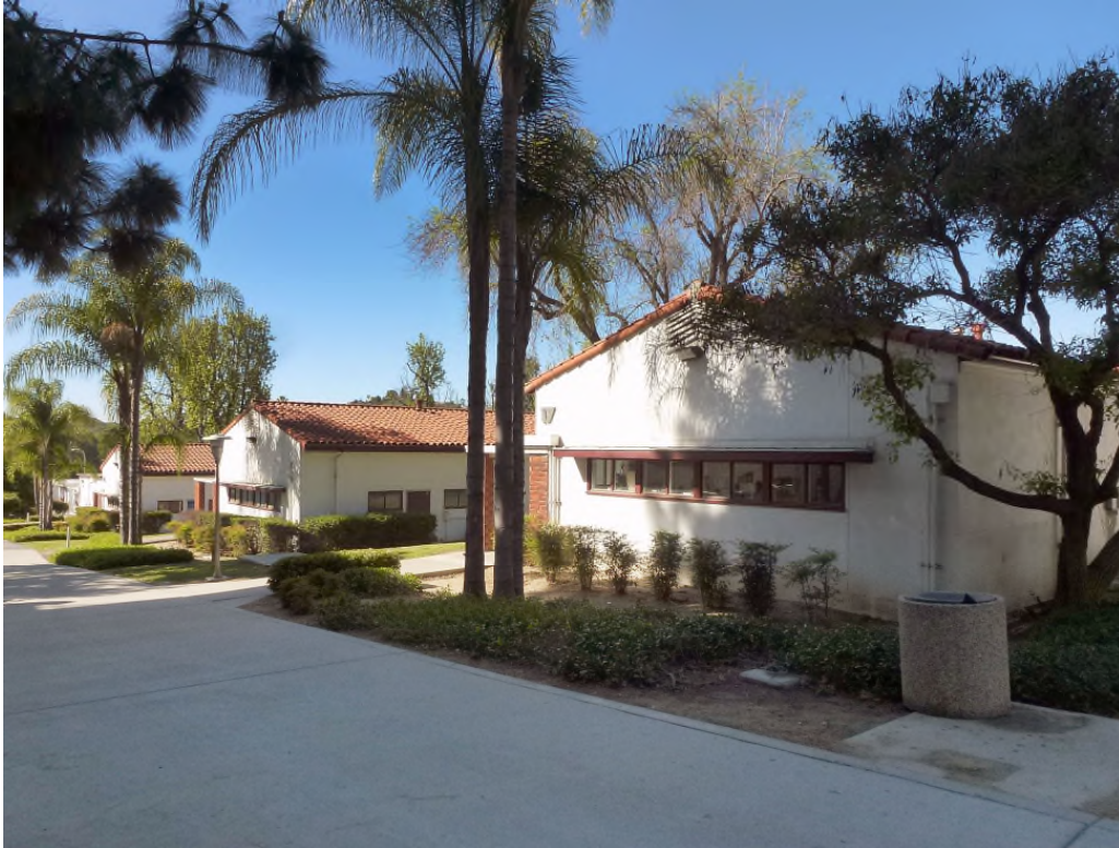
Figure 39. Oblique of east and north façades of Buildings 17, 18, 19.
