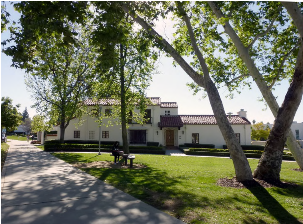
Figure 38. View of the west façade of Building 10.
