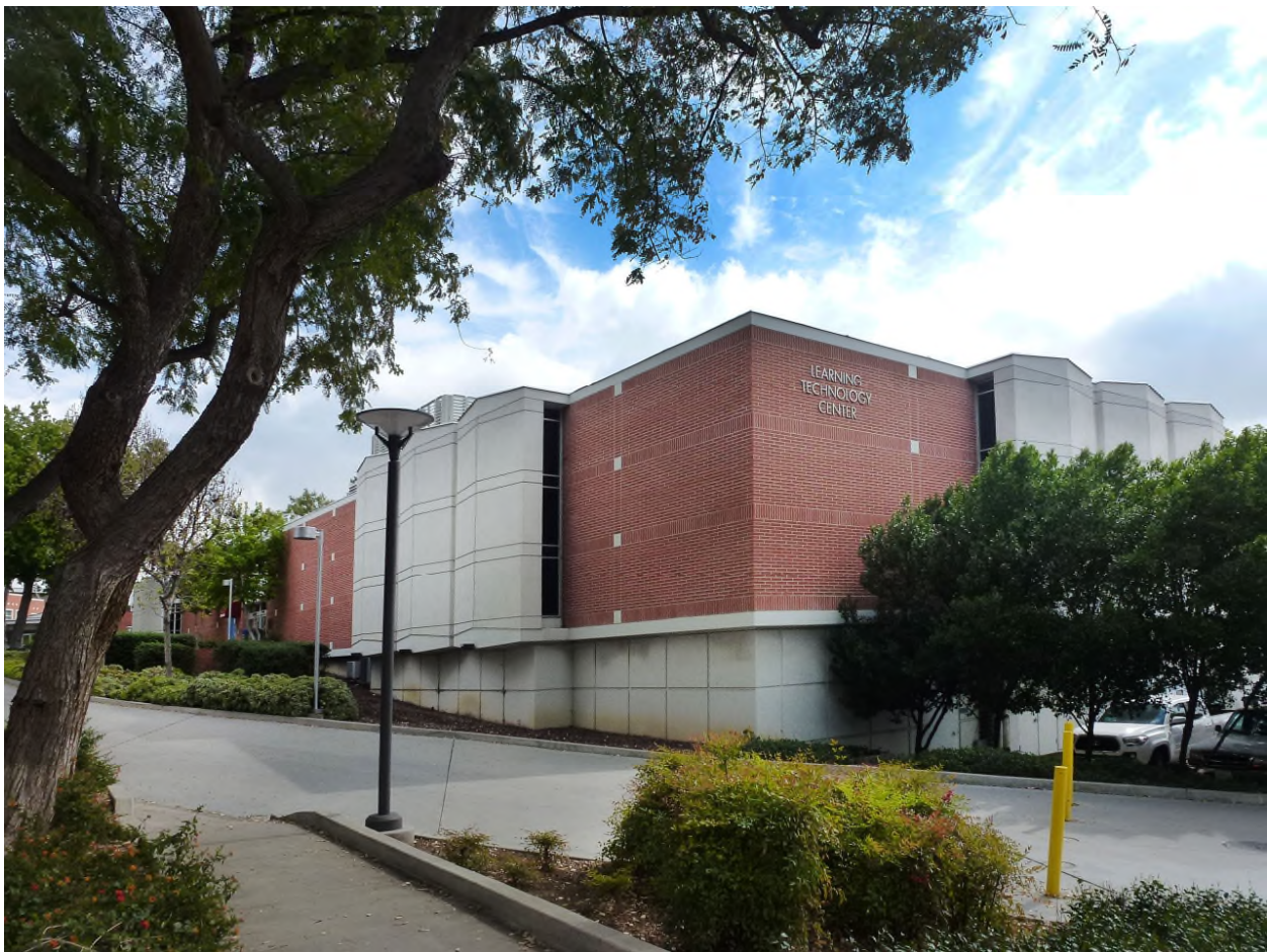
Figure 14. Oblique view of the north and west façades of Building 6.
