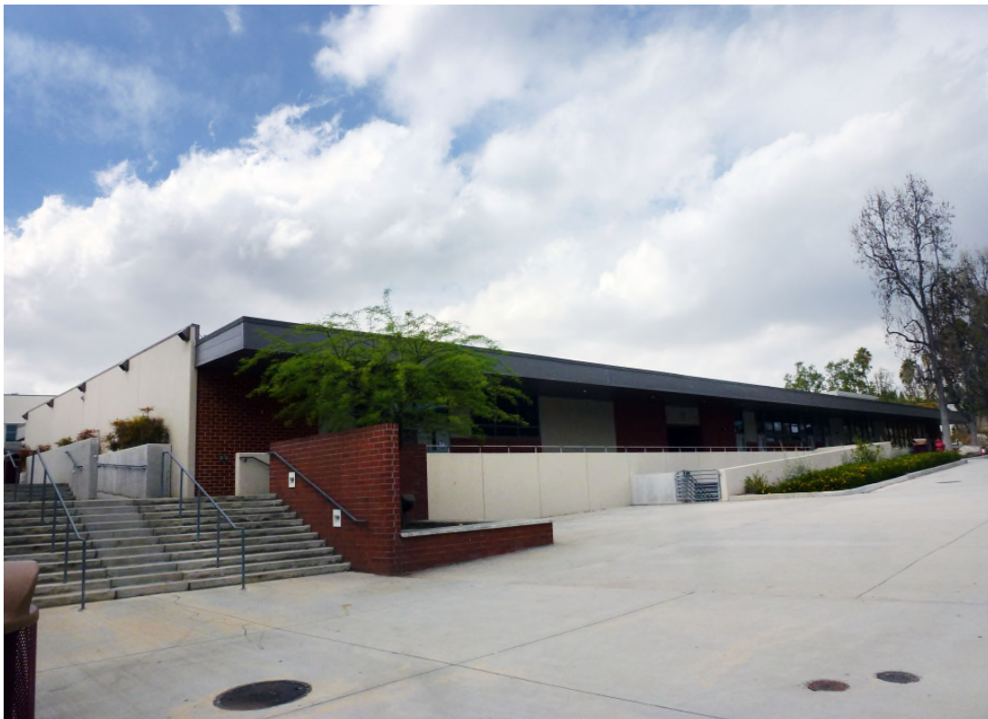
Figure 17. Oblique view of the east and south façades of Building 11.
