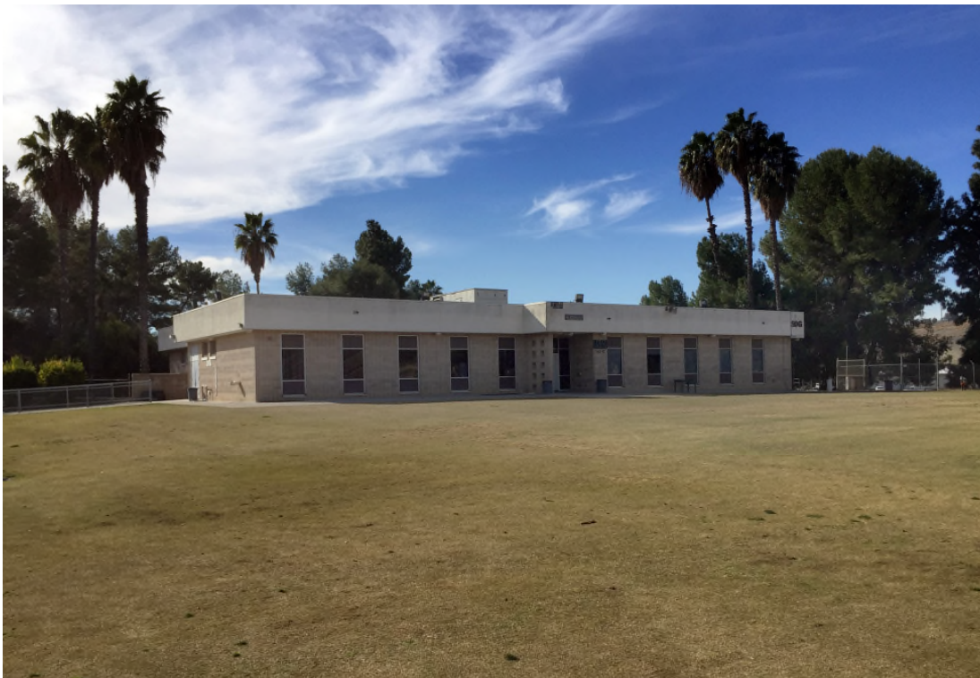
Figure 8. Field House (50G), view looking southeast of east and north façades.
