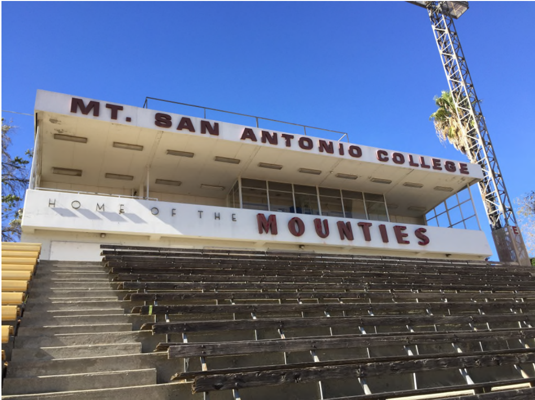
Figure 7. Press box (50F), view looking west of east façade.
