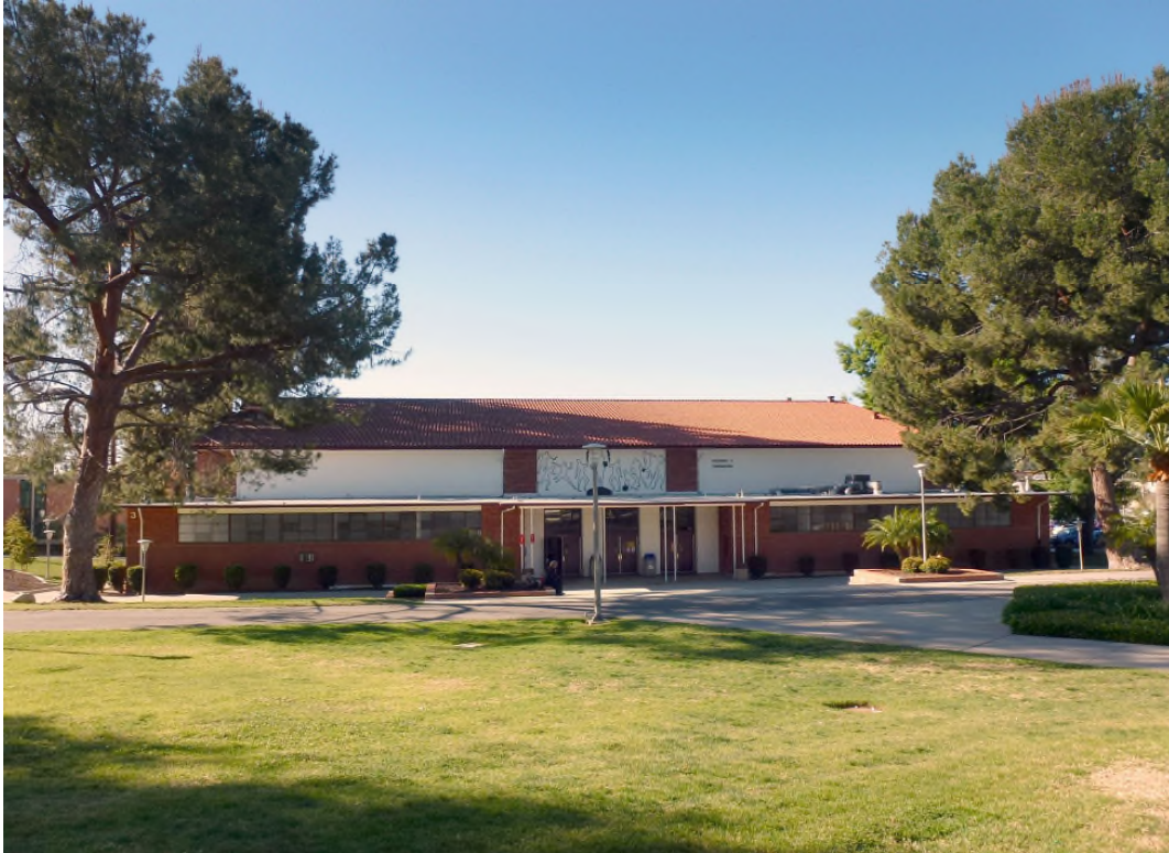
Figure 37. Primary (north façade) of Building 3.
