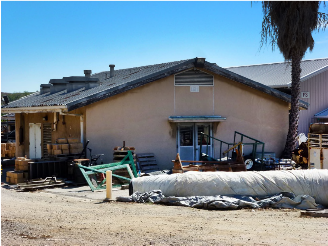
Figure 29. Oblique view of the north and west façades of Building F3A.
