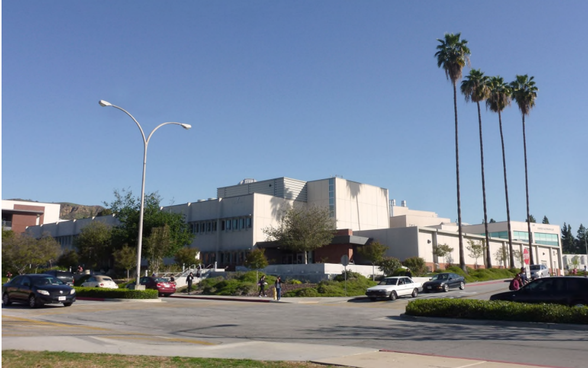
Figure 15. Oblique view of the west and south façades of Building 7.
