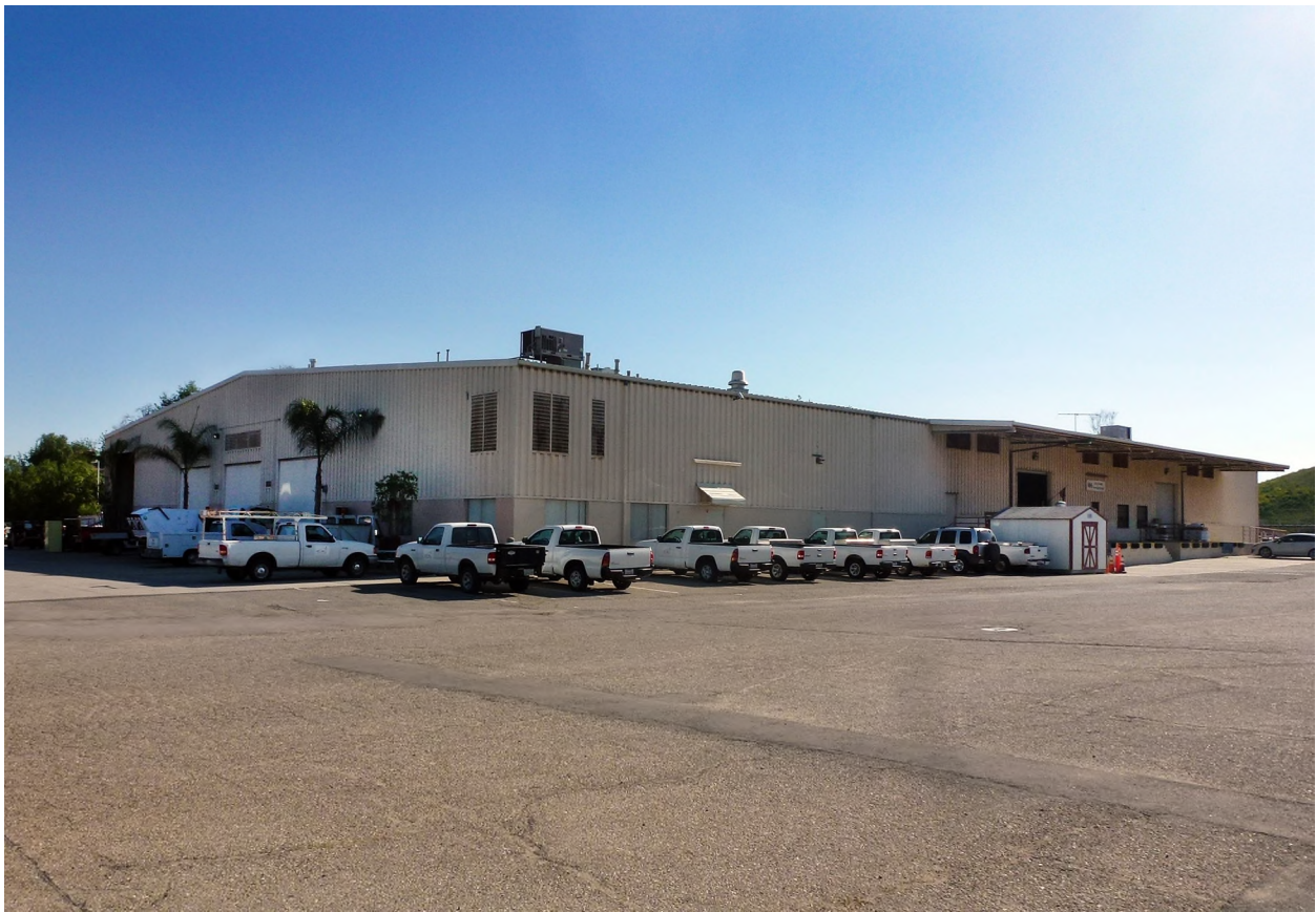
Figure 25. Oblique view toward the south of the northwest and northeast façades of Building 48.
