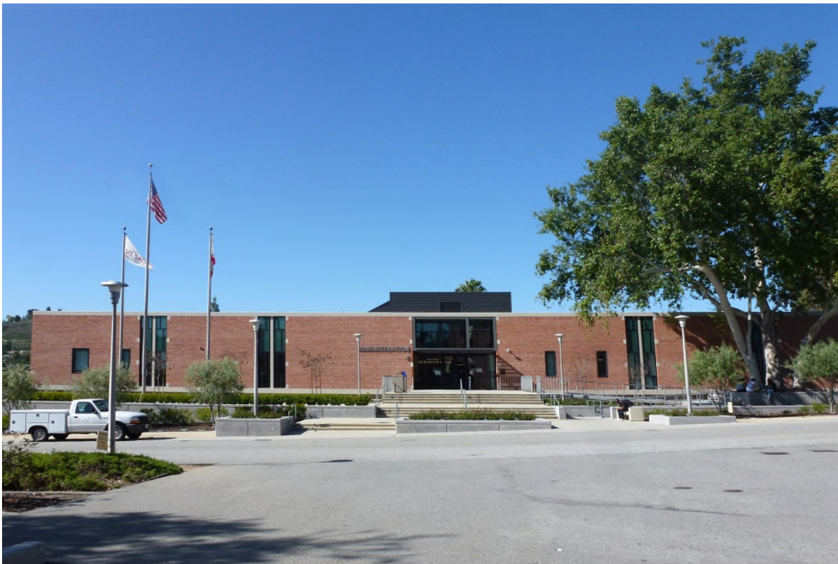
Figure 13. View of the primary (west) façade of Building 4.
