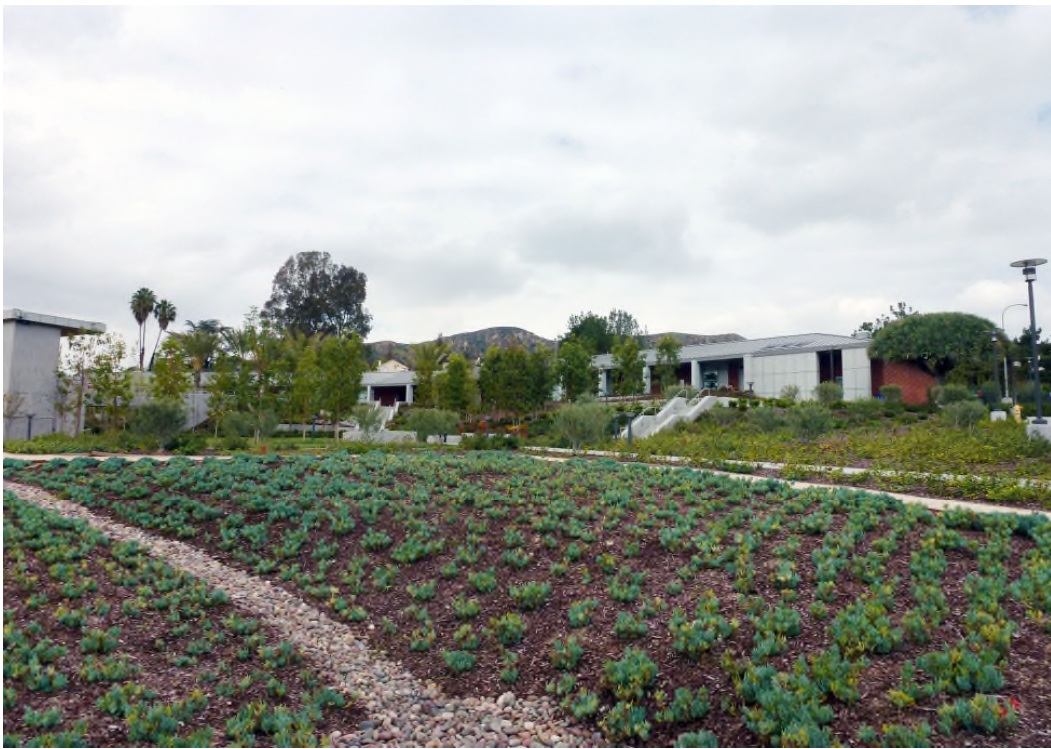
Figure 18. View of the south façade of Building 12.
