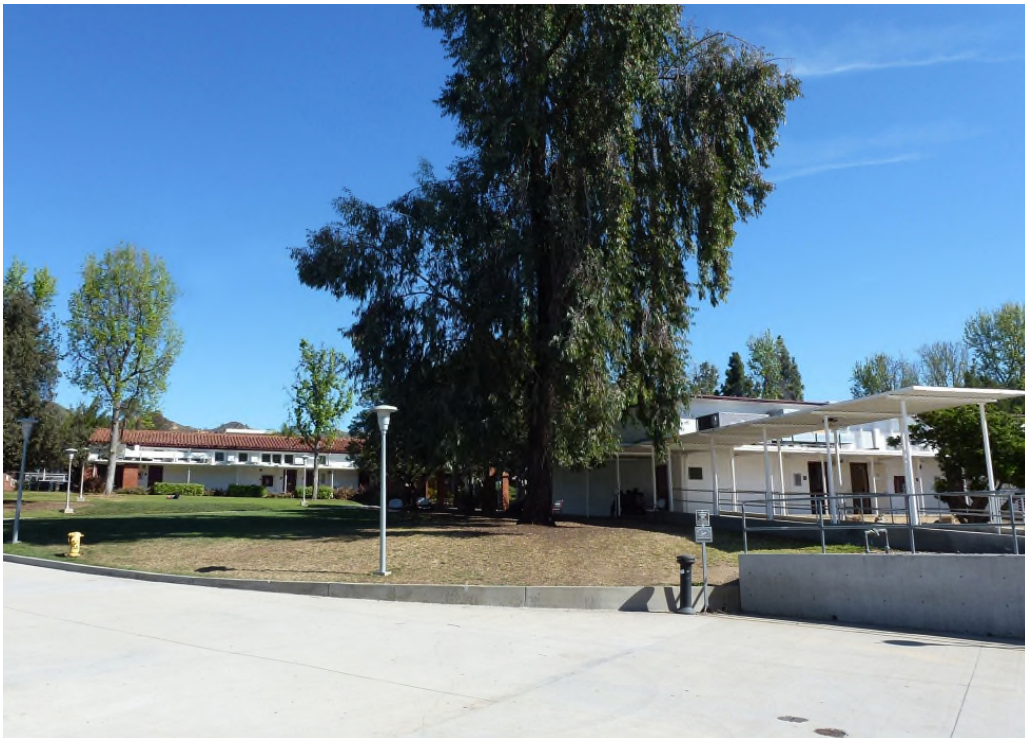
Figure 40. Oblique view of the west and south façades of Building 20. Building 18 is to the left of the photo.
