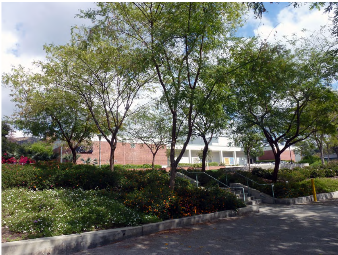
Figure 12. View of the south façade of Building 1A.
