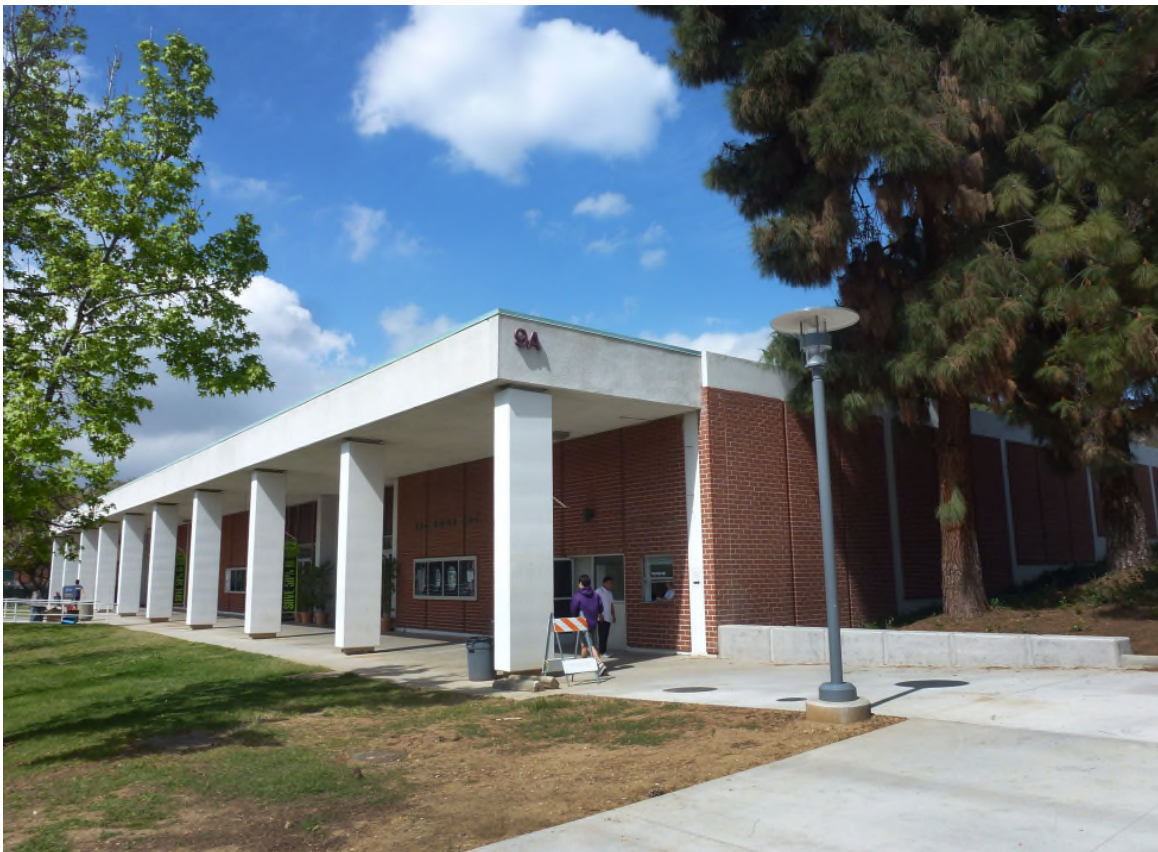
Figure 16. Oblique view of the south and east façades of Building 9A.
