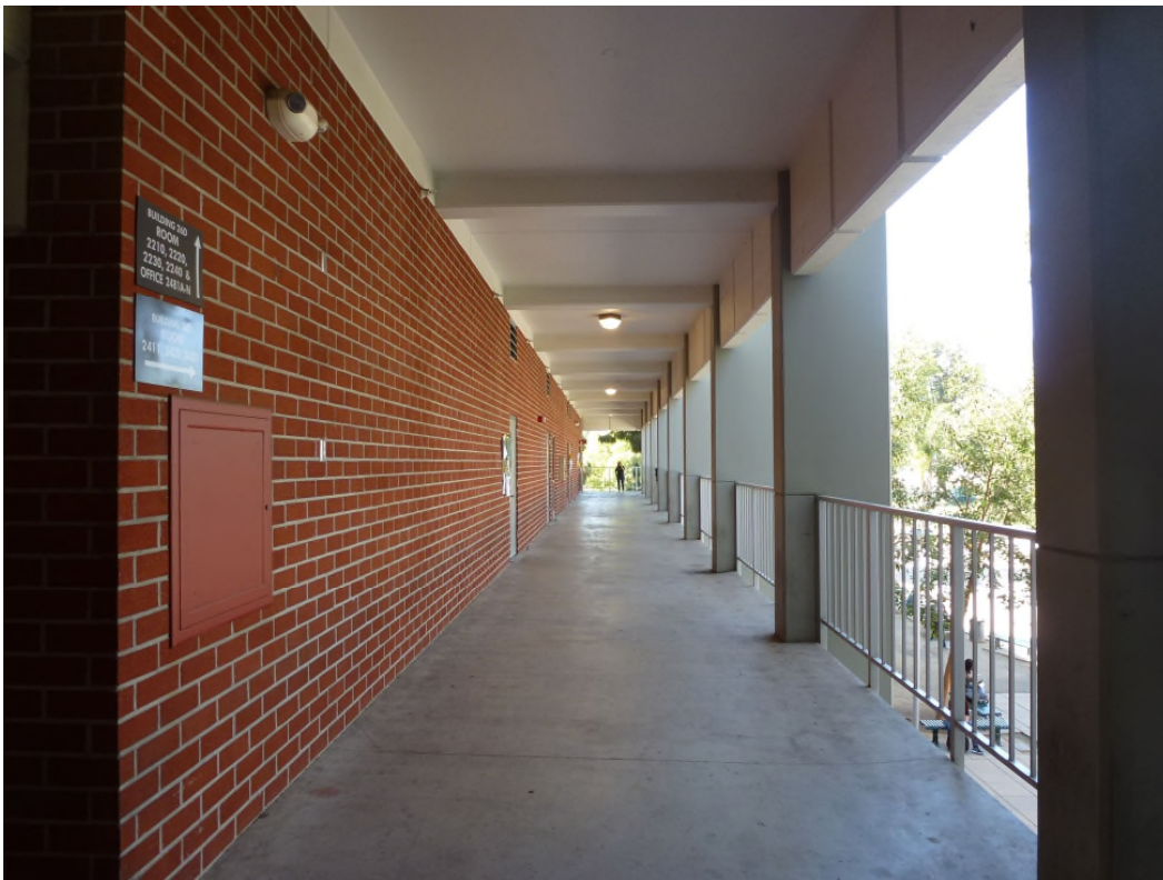
Figure 21. View of the second story corridor of Building 26D.
